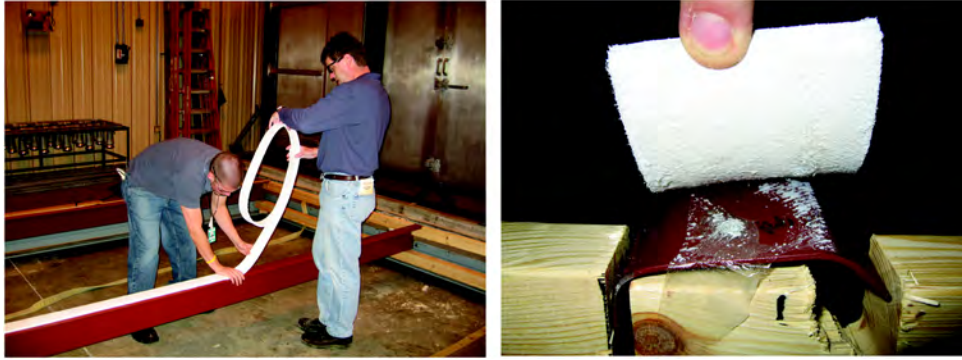
Figure 5 Installation of the aerogel strips on top of the steel purlins.
